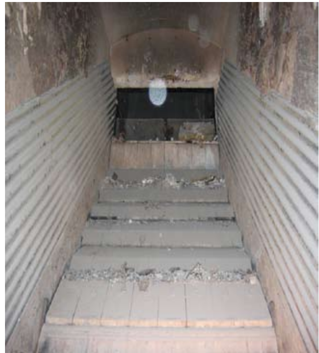
Rebuilt plant in Torshavn. The plant has a capacity of 2 t/h and is shown here after 4000 hours of operation.
