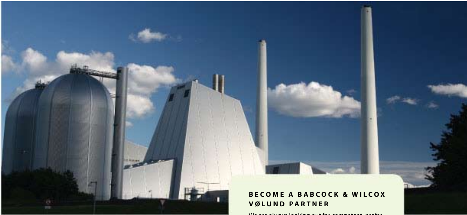
Avedøre CHP plant, Denmark – the world's largest straw-fired supercritical boiler
