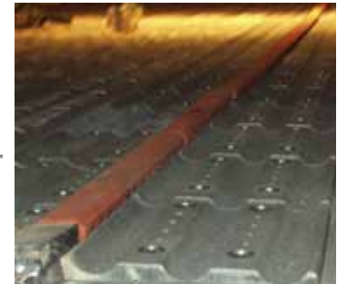
Cast iron plates to be placed on top of the tubes of the vibrating grate.
