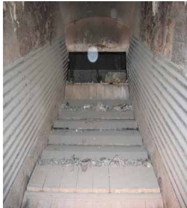
Rebuilt plant in Torshavn. The plant has a capacity of 2 t/h and is shown here after 4000 hours of operation.
