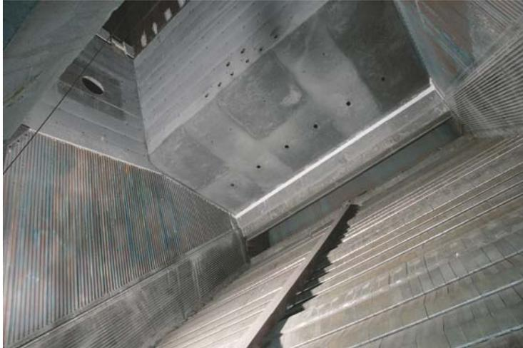
Figure 9: Combustion chamber with central-flow firing
